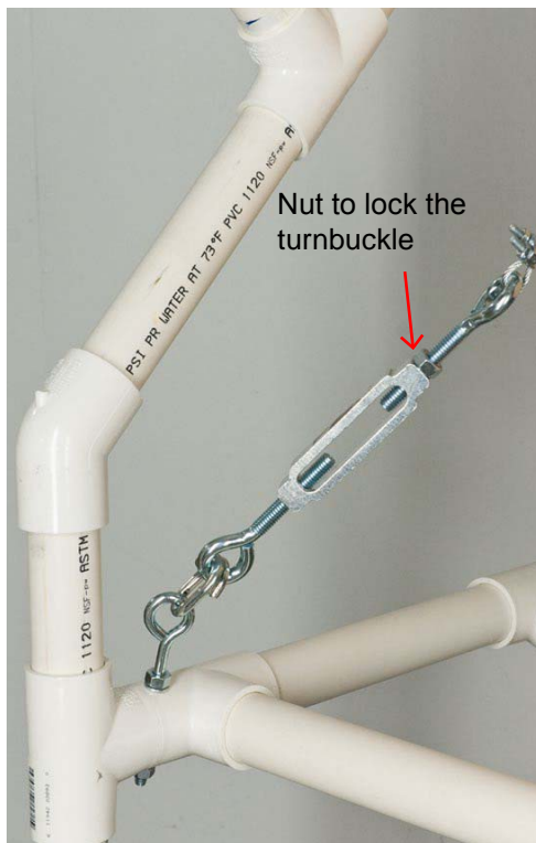
Figure 57 Drill a hole for the eyebolt. Install the cable. Adjust the turnbuckle so that the table top is perfectly vertical when in the upright, "photo" position.
