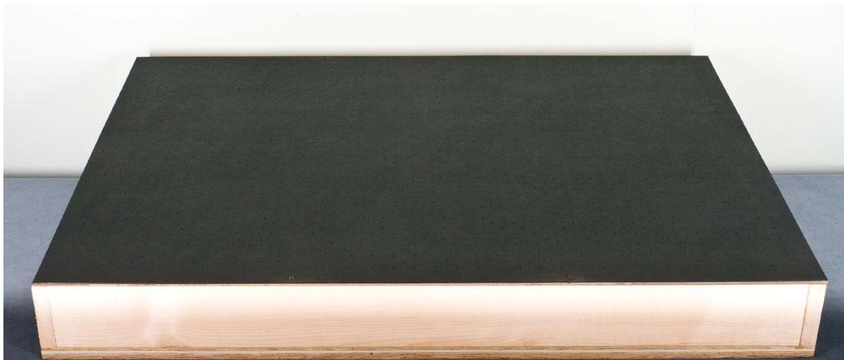
Figure 39 After screwing the hardboard in place, screw the black plastic on top. This completes the table top.
